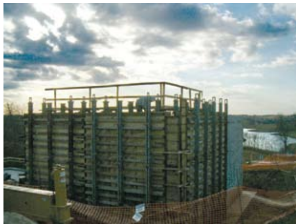
Design/build by BCI for pre-treatment plant additions for Nestle Prepared Foods.
