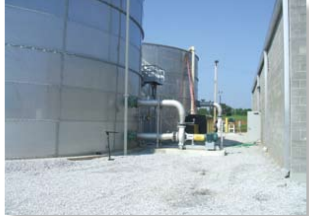
Outside Aeration Tanks
