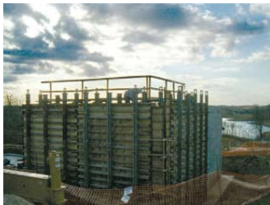
Design/build by BCI for pre-treatment plant additions for Nestle Prepared Foods.
