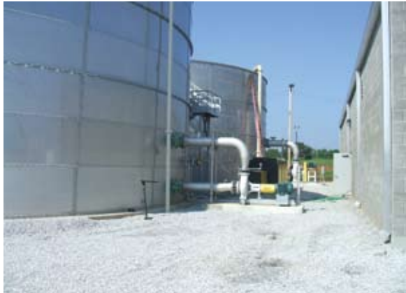
Outside Aeration Tanks
