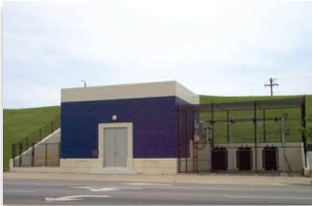
Northern Kentucky Sanitation District 1 Storm Water Pump Stations Upgrade
