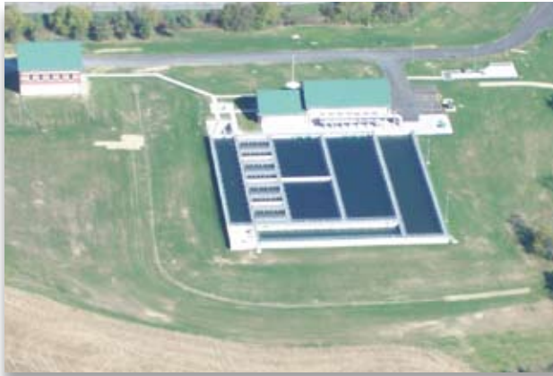
Town of Plainfield, South Wastewater Treatment Plant
